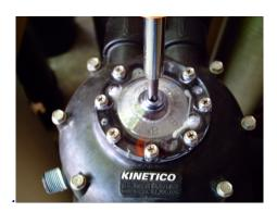
4. Firmly push the screwdriver straight down until it stops. Then slowly turn it clockwise (right). This will rotate a small disk about the size of a dime which has a wedge shaped protrusion on it. Shown below near the tip of the screwdriver just below the word "Brine."
